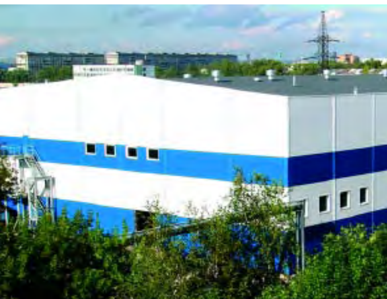
New autocatalyst manufacturing facility in Krasnoyarsk, Russian Federation.
