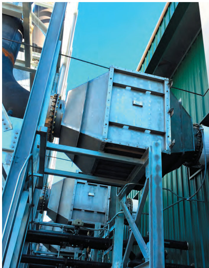
Johnson Matthey's emission control system with SCR, ASC and oxidation catalysts in a single, compact housing.
