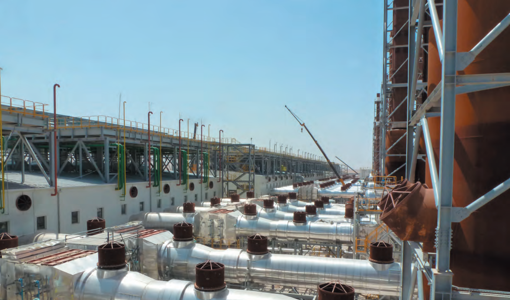
Middle East power plant operating thirty-eight 17 MW, HFO-fueled engines, each one equipped with a Johnson Matthey SCR system.
