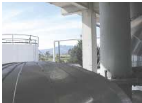
The Interquimec plant (elevation 3050 meters) with volcanic mountains in the background.
