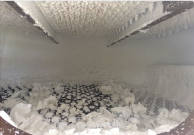
Figure 2: Inside of UFC absorber where solids have formed
