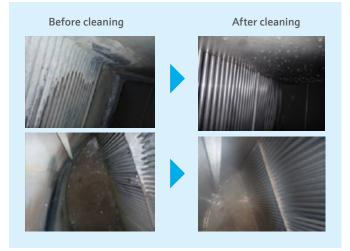
Figure 3: Vaporizer - before and after cleaning
