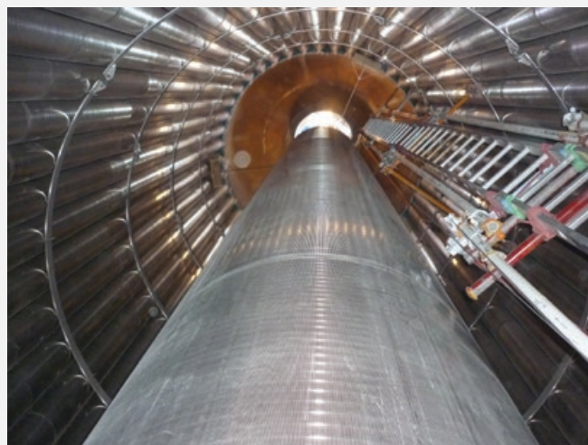
Inside a JM radial flow reactor
