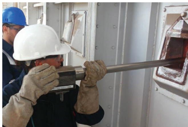
Above: Thermal footage is recorded at every peephole.
