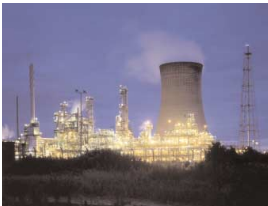
BP Chemicals' plant at Hull, UK has an annual capacity of 250,000 tonnes vinyl acetate monomer
