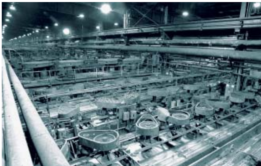
Banks of flotation cells at Norilsk Nickel's Talnakh operation on the Taimyr Peninsula in Siberia.
