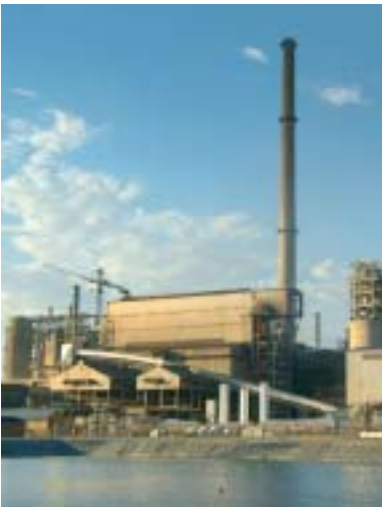
A new, higher capacity converting process plant, which will substantially reduce sulphur dioxide emissions, and a slag cleaning furnace were commissioned at Anglo Platinum's Waterval Smelter in 2003.
