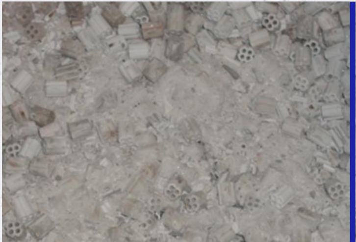
Severe fouling of main bed
