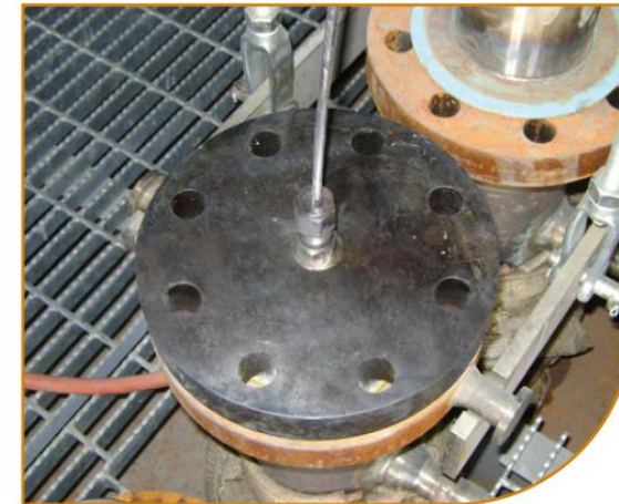
CatTracker installed in a reformer tube
